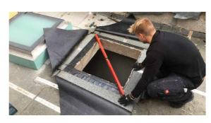
**Step 4.**Marking the outer edge of the Skyfloor/insulation frame for an uniform alignment.
